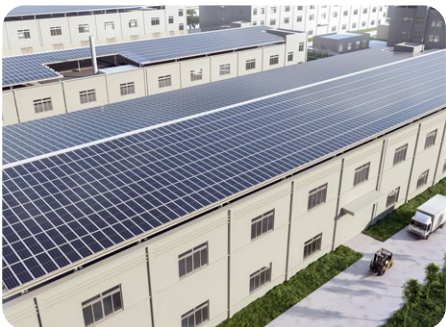
Flat-to-pitched Roof Conversion
