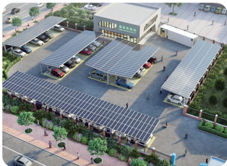
PV Charging Carport With Storage
